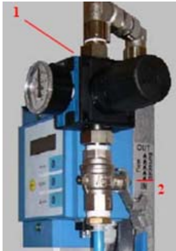
Output installation: [1] Regulator with manometer [2] 8 mm tube / 1/2" fitting
